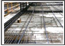
(iv) the provision of minimum longitudinal steel (untensioned reinforcement) at column positions for all flat slabs of at least 0.075% of the gross concrete cross-sectional area, concentrated between lines that are 1.5 times the slab depth either side of the width of the column and extending 0.2L into the span, L [cl.6.10.6 TR.43]
